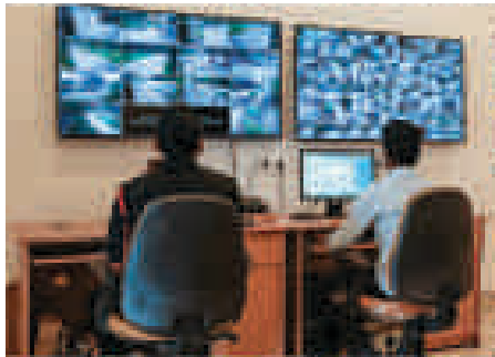
CCTV Control Room
